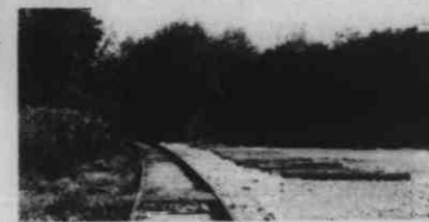
A railroad siding comes to Keystone's 15 acre site.
